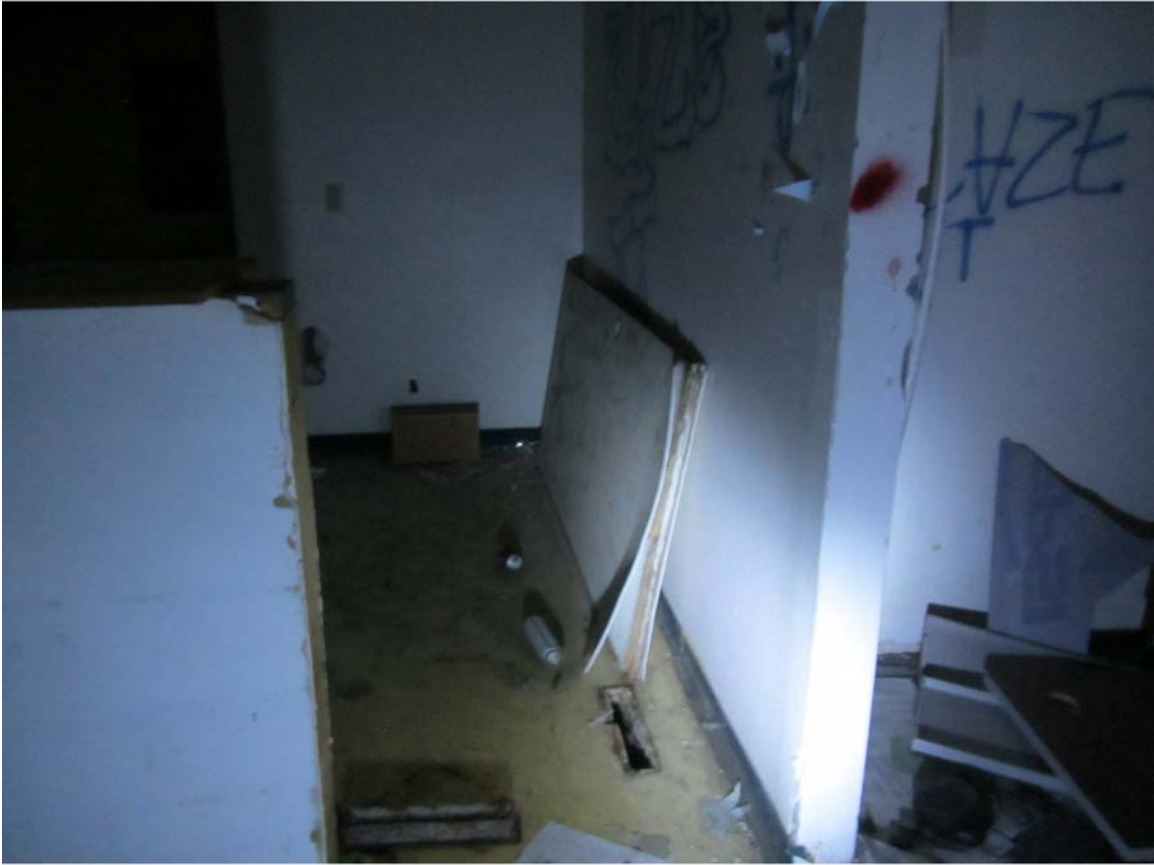
Photo 33 - Interior of a Door Exposed. No Suspect ACM
