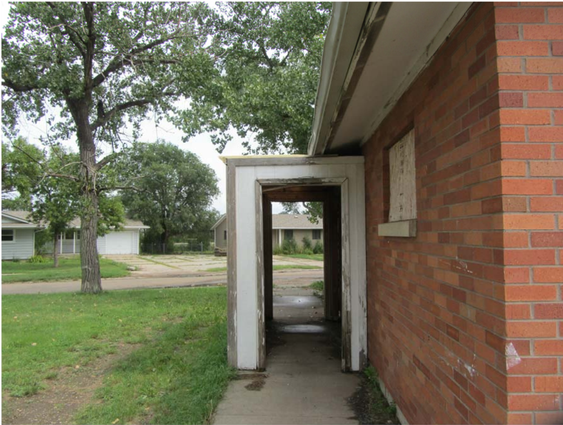
Photo 3 - North side of the Building and Suspect Front Entry
