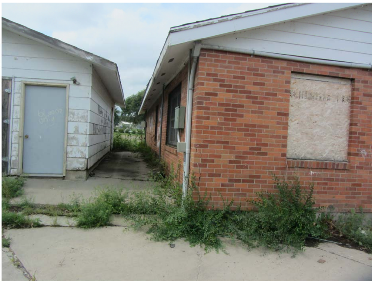
Photo 6 - South Side of the Building
