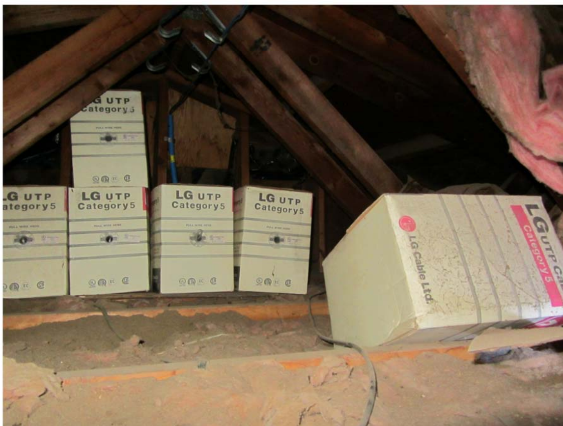
Photo 16 - Boxes Being Stored in Attic. Forgotten Files?
