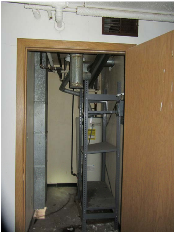
Photo 18 - Hot Water Heater And Some Mechanical Piping Included Muddled Fittings
