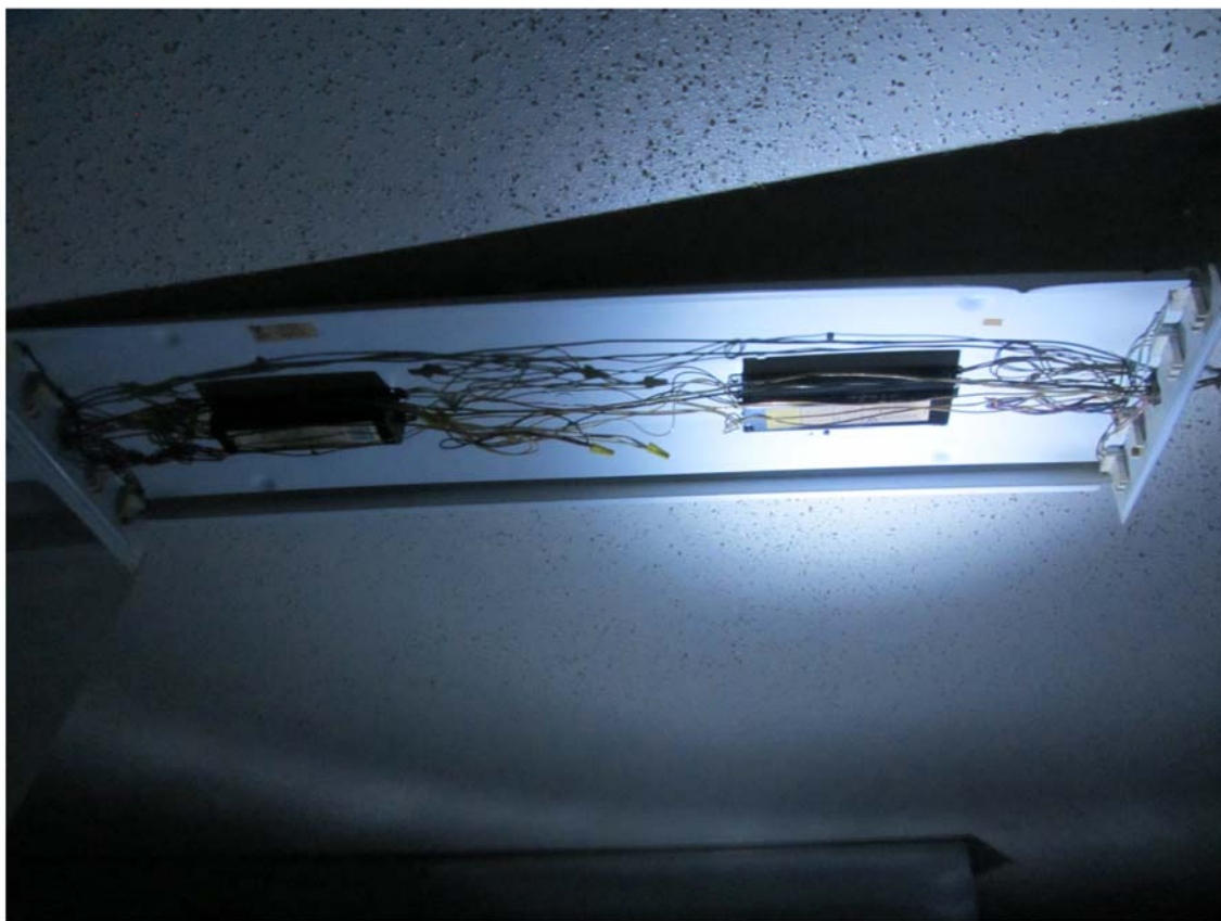
Photo 27 - Fluorescent Light Ballasts
