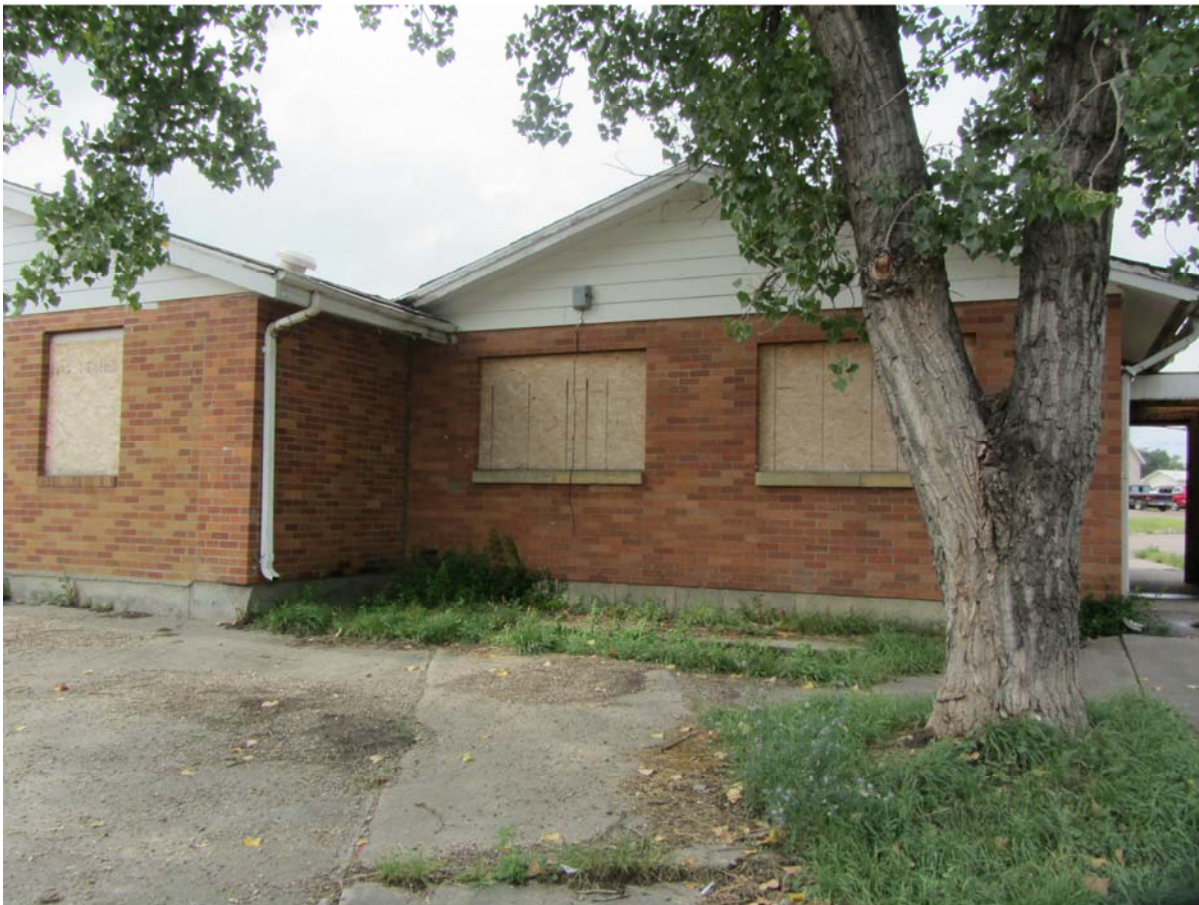
Photo 5 - East Side of the Building
