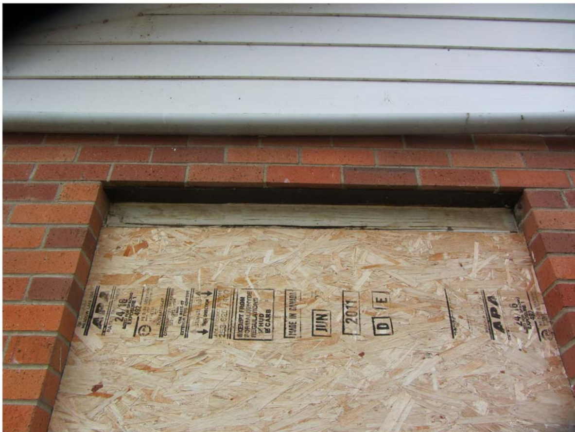
Photo 12 - Another View of Window Blanking
