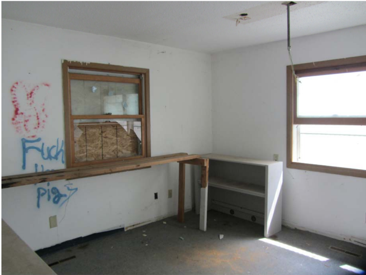
Photo 19 - Southeast Office Area
