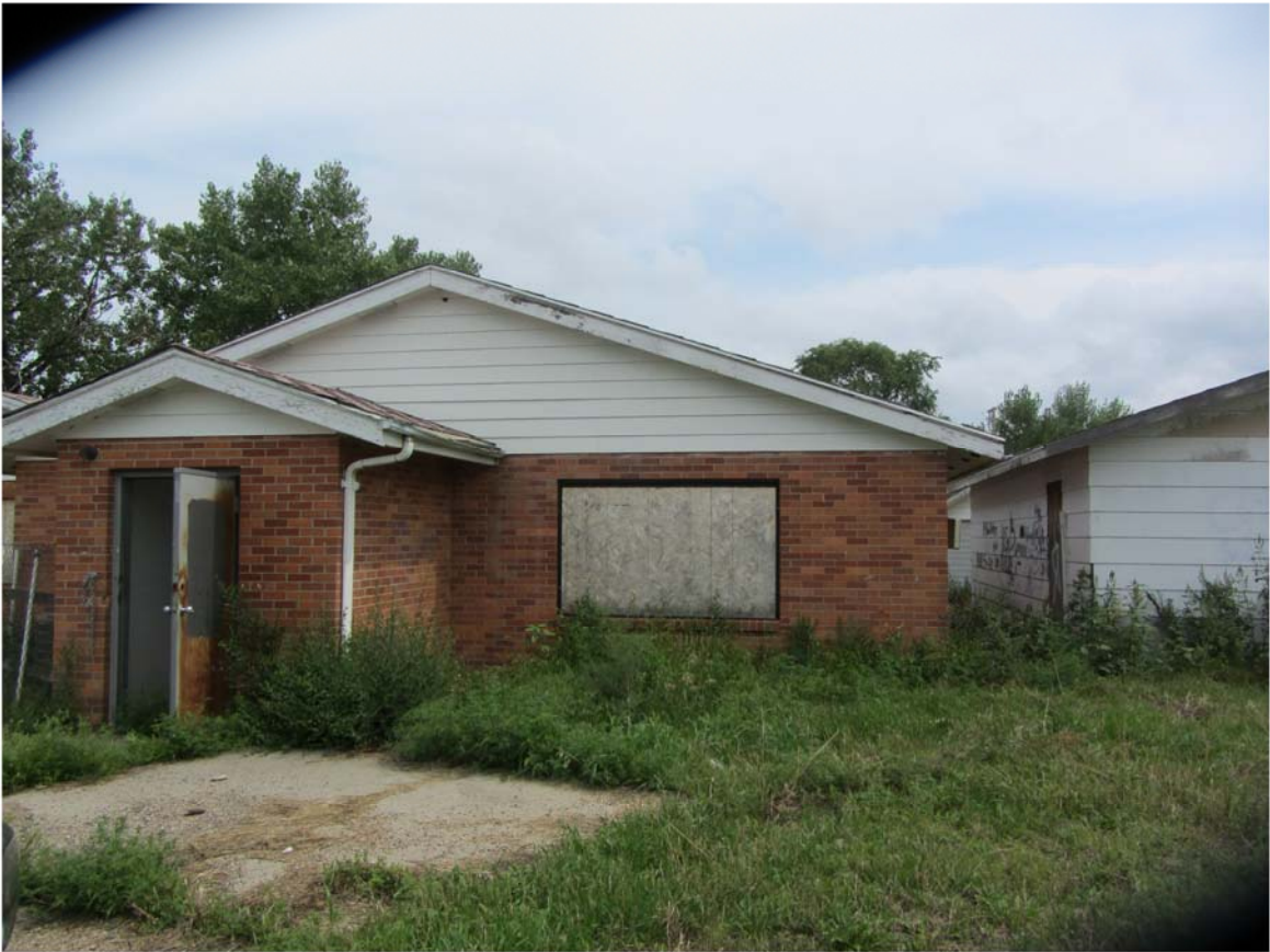
Photo 1 - West Side of the Bldg and an Entry Point
