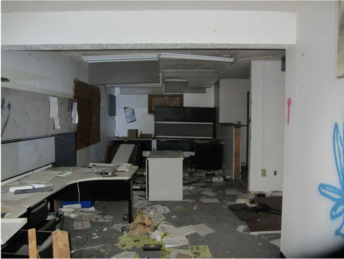
Photo 21 - View of the Building Looking From the South to the North
