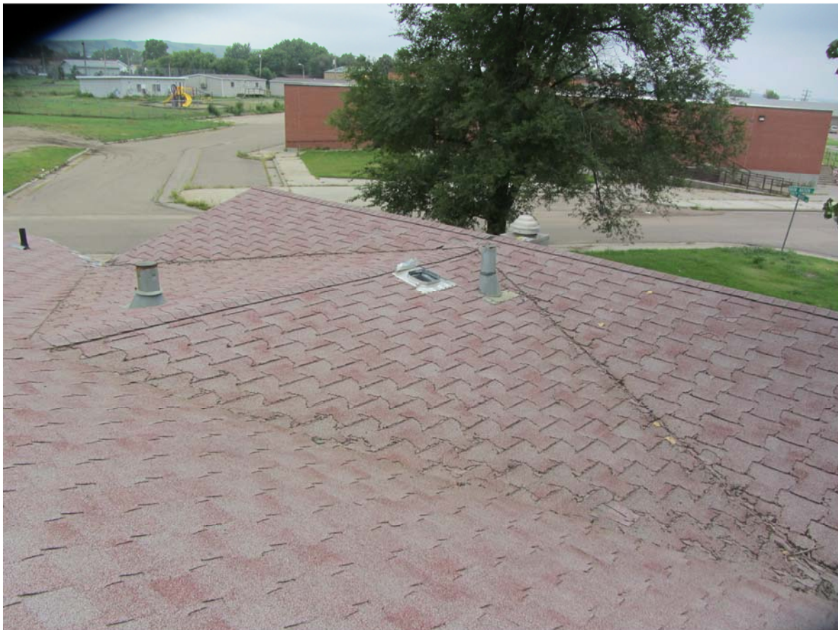
Photo 9 - Roof Showing Some of the Mechanical Penetrations
