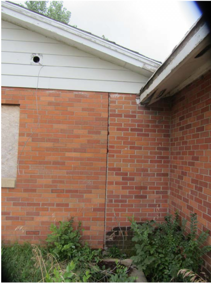
Photo 13 - Sealant Between the South and North Building Sections. Roof Fascia and Trim Boards Are Painted
