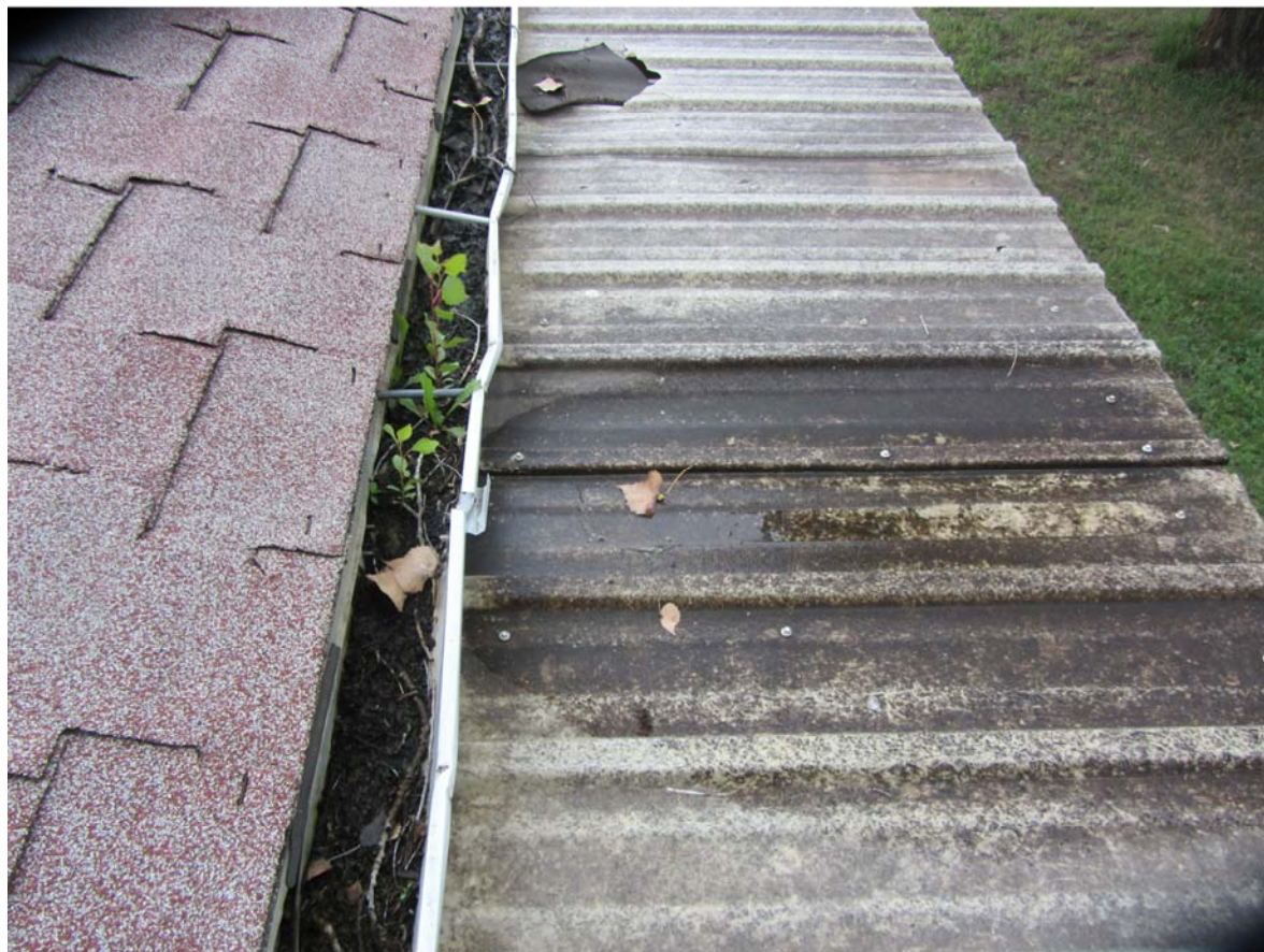
Photo 7 - Open Air Entry is Fiberglass and Roof is Fiberglass
