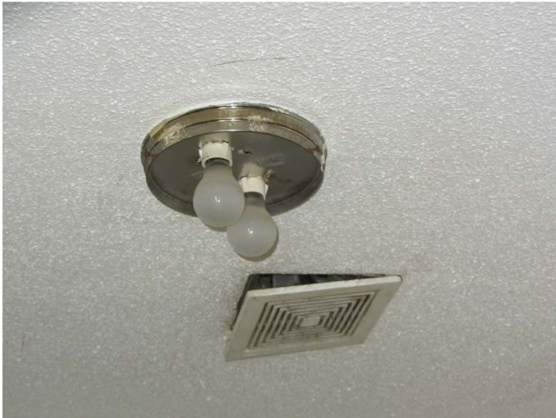
Photo 23 - Ceiling Texture is Throughout the Building. This Material is ACM
