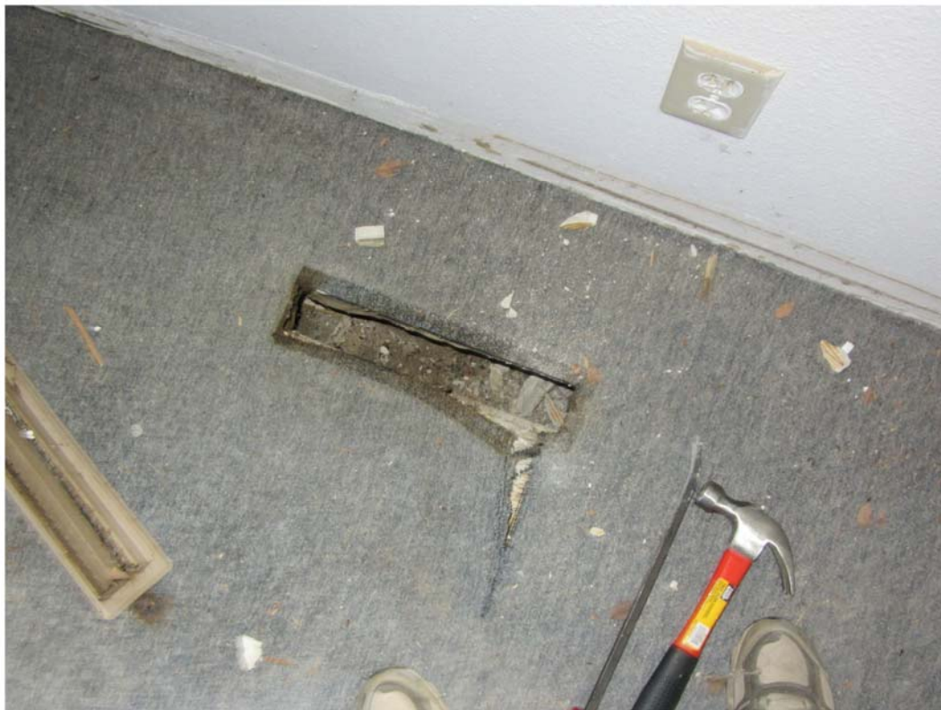
Photo 32 - Underfloor Supply Duct Work
