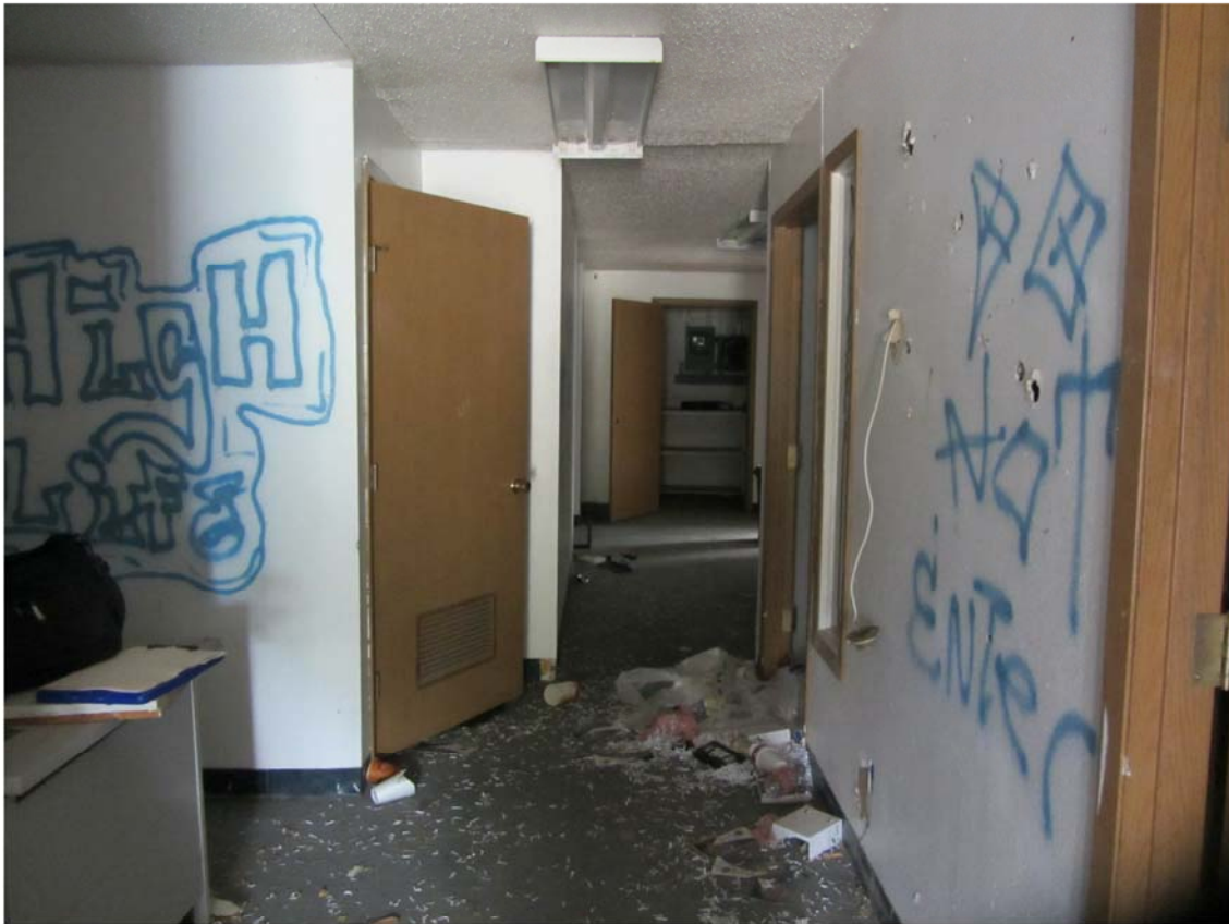
Photo 17 - Interior of the Building General View
