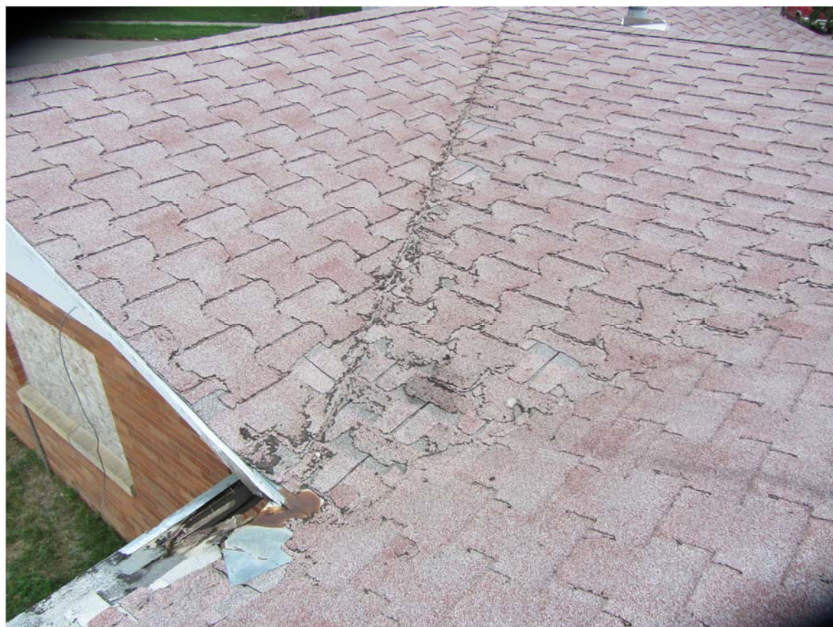
Photo 8 - Building is Asphalt Shingled with Multiple Layers
