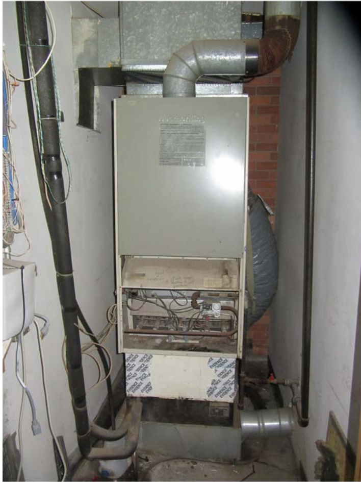
Photo 31 - Building Forced Air Furnace
