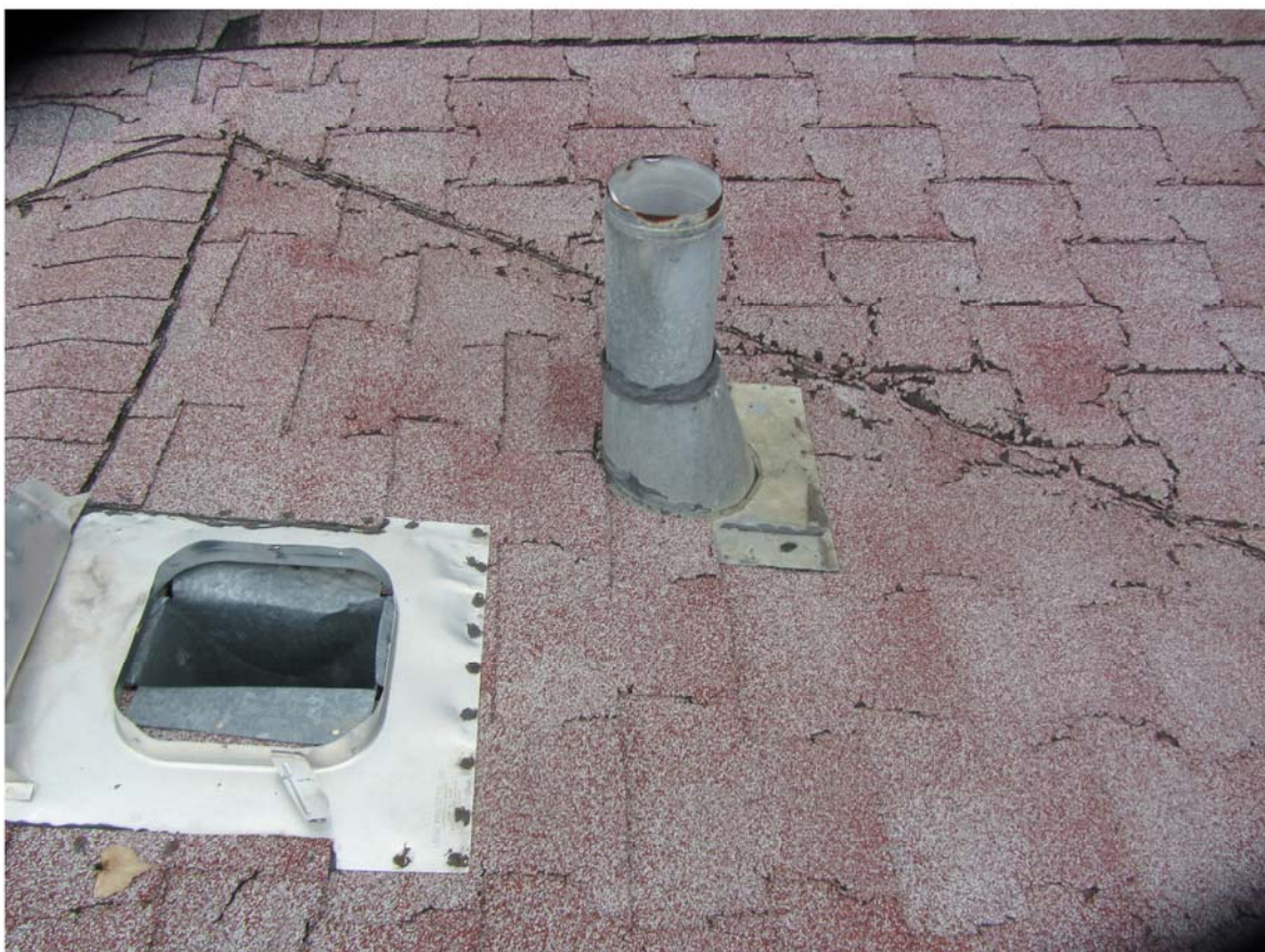
Photo 10 - Penetrations with black Sealant that is ACM
