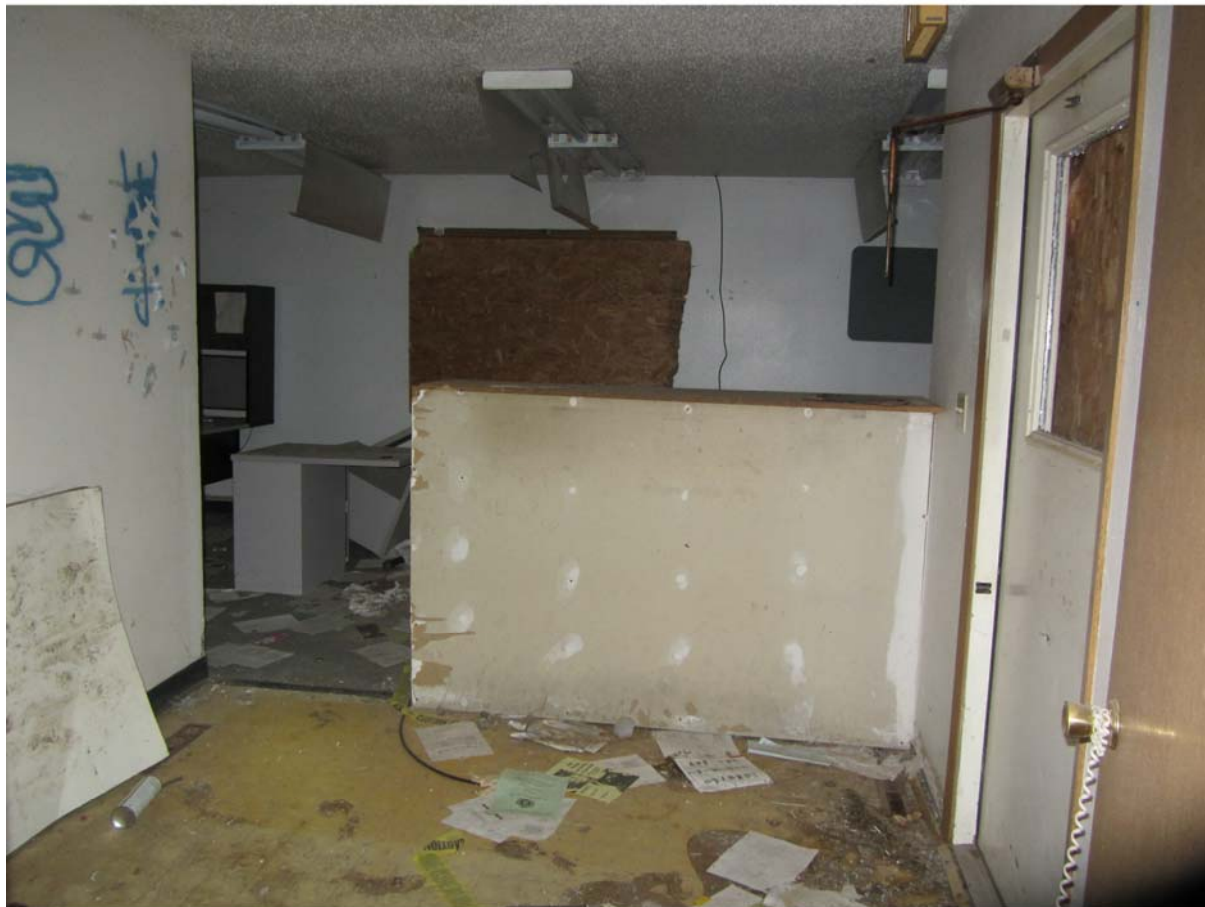
Photo 20 - Looking North Into North Building Section
