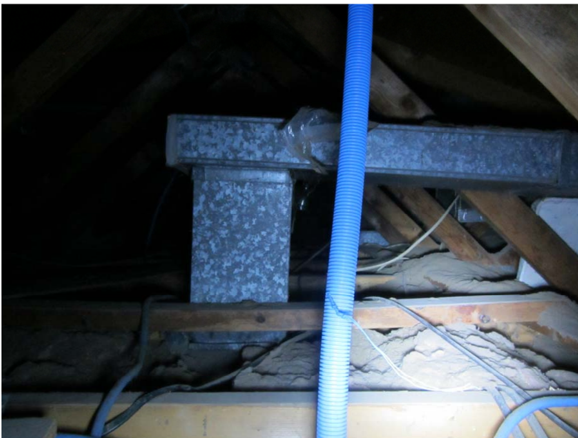
Photo 15 - Attic Area. A Layer of Fiberglass Bat Insulation is All That is Present
