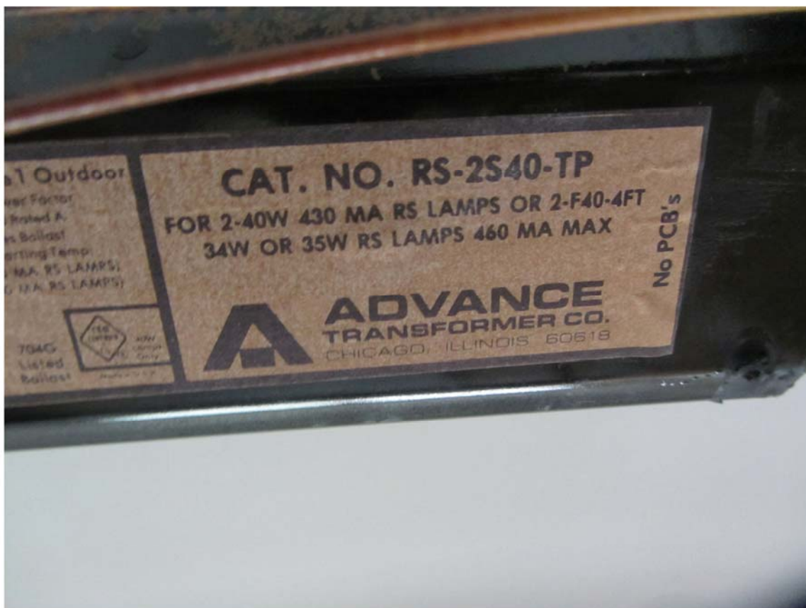
Photo 28 - Close Up of Ballast Showing "No PCBs" Label
