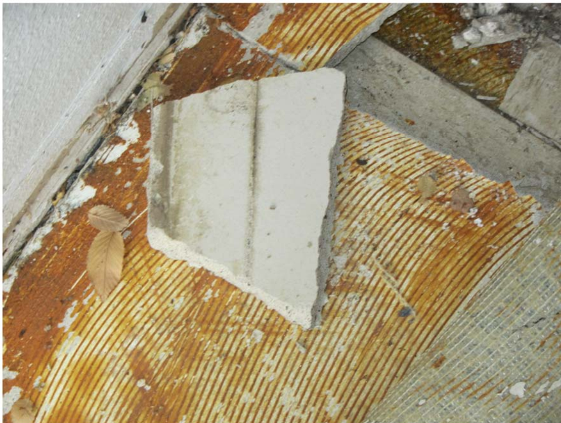
Photo 24 - Flooring System is slab on Grade, Vinyl Floor tile, Thick Leveling compound And Carpet or Sheet Vinyl in Most Areas. Bottom Most Vinyl Floor tile Seemed to only be In Restrooms, and Office in the Main Section of the Building.
