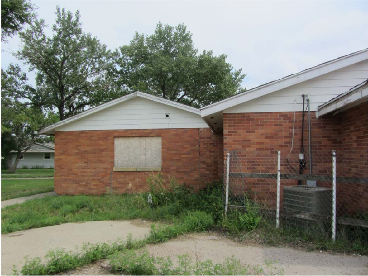
Photo 2 - West Side of the Bldg Showing AC Compressor Slated to be Moved and North Section
