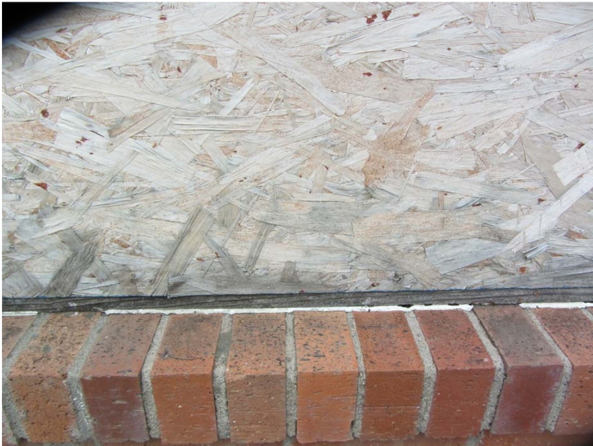
Photo 11 - Window Blanking Sealant
